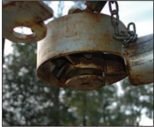
The simple pipe-gate design with a 6-lock system.
