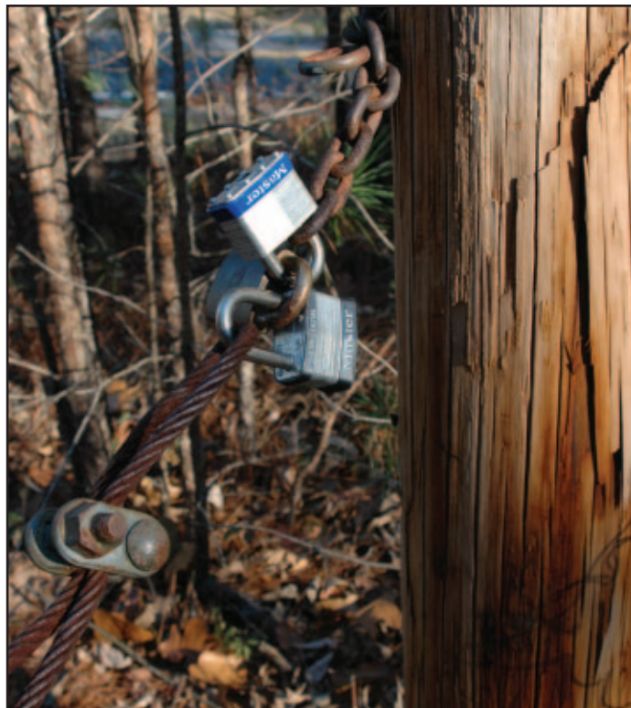
Utilizing a chain locking system allows for easy bolt cutter access to locks and chain links. In addition, others can cut chain links and incorporate their lock onto the gate.
