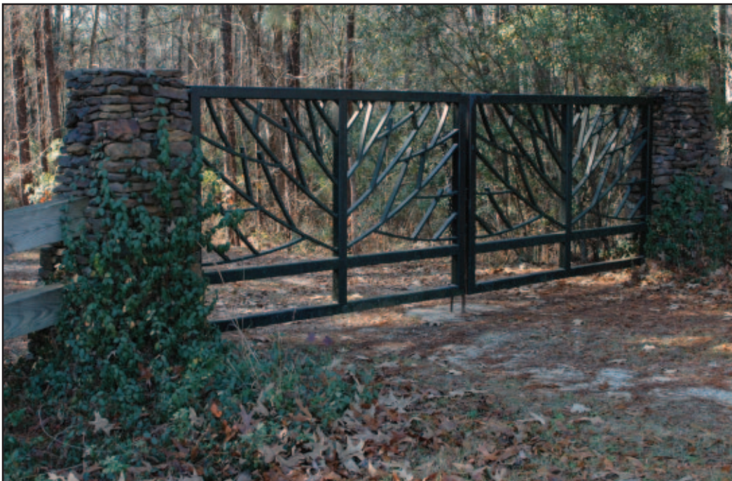
A good example of a custom fabricated heavy-duty gate that has utilized native rock to veneer the concrete posts in order to allow the gate to better blend into the surroundings
