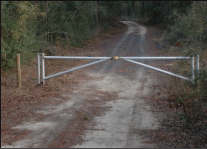
A basic pipe-gate design positioned to prohibit vehicles from circumventing the gate.
