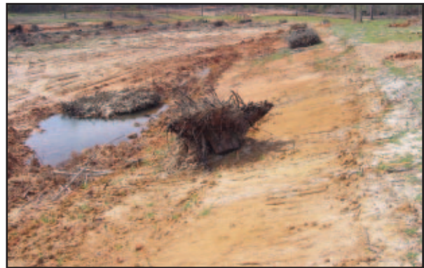
Use of entire tree to make good structure along shoreline
