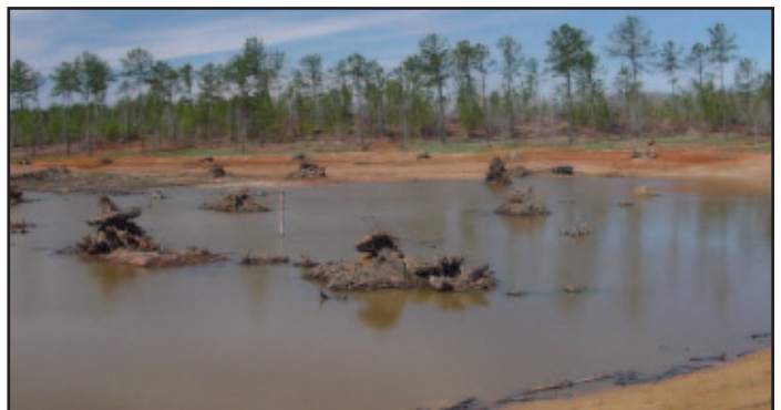
Heavy equipment used to install large structure in pond
