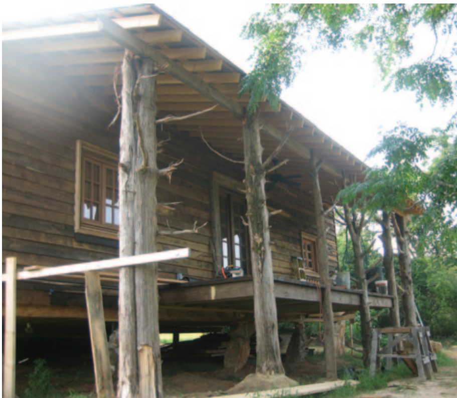
Reclaimed fallen cedar trees from the farm used as porch columns.
