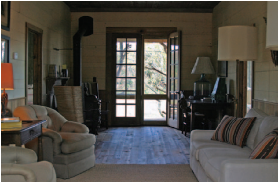
Reclaimed Heart Pine floors, Sinker Cypress Wainscot and lime painted 1x6, 1x8 New Pine wall board and ceiling. Please note wood burning stove in lieu of masonry fireplace.
