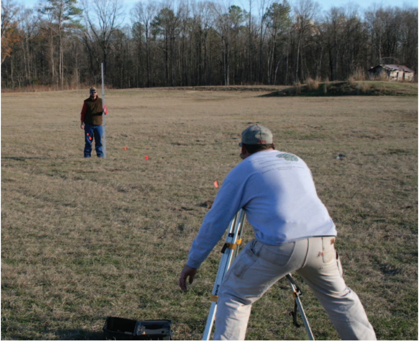
Surveying the land and flagging the shoreline can give you an idea of the size and how the lake will lay out.
