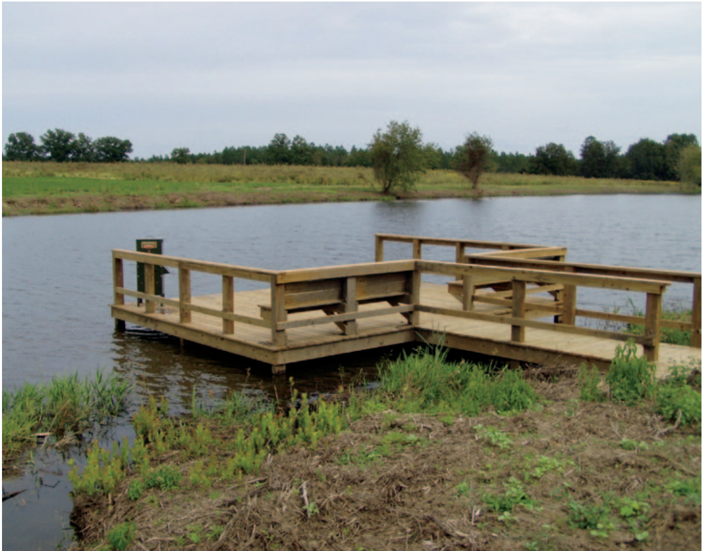
This dock is fairly simple yet functional with a fish feeder added to it. The feeder was angled to throw feed across in front of the dock rather straight out from one side or the other. No railing in front allows for easy fishing, docking a small boat, or diving in on a warm summer day. Fish attractors could be placed on both sides near or out from shore to provide habitat for fish.
