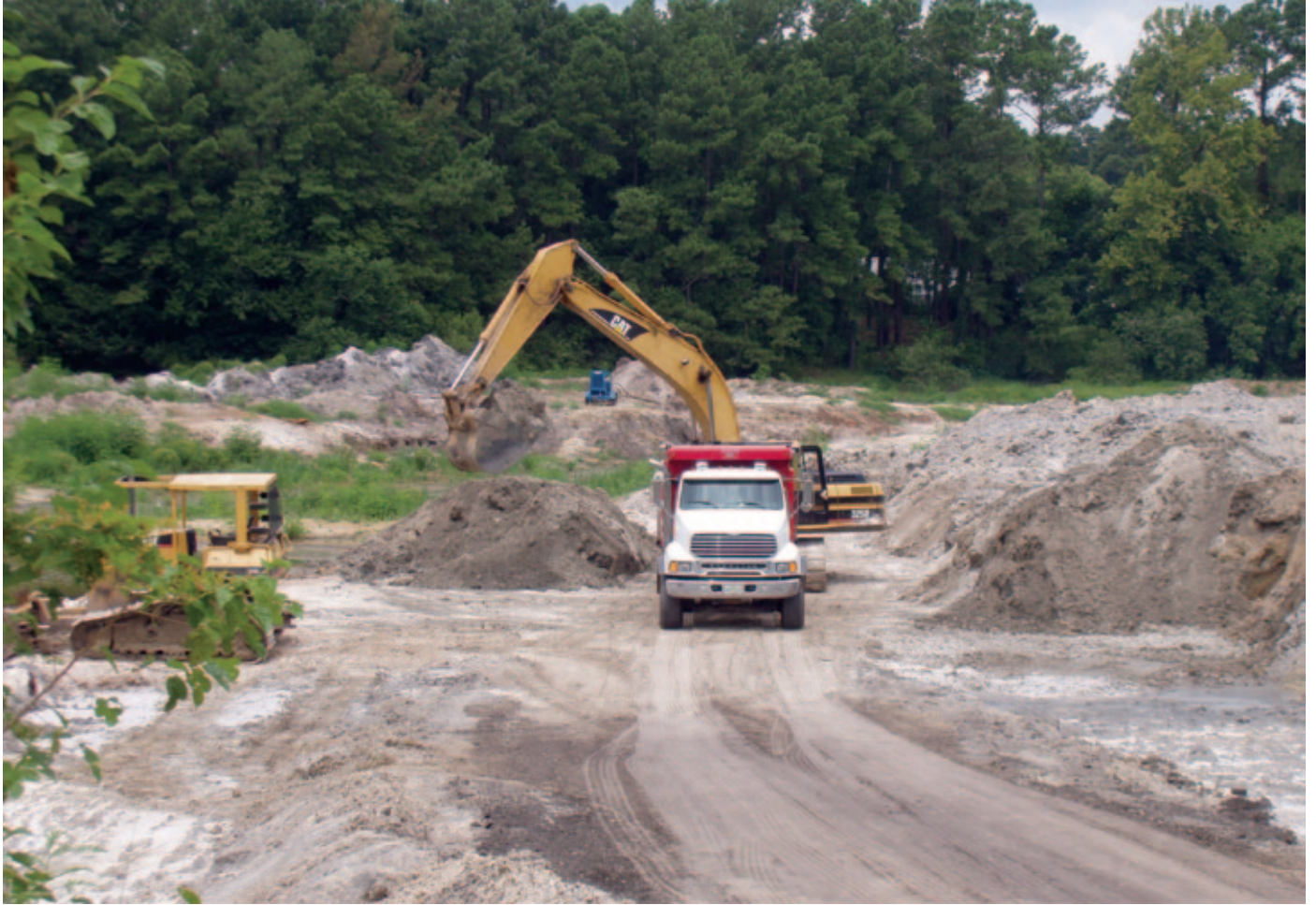
Some draw downs are simple, but this one entailed drawing down, scraping out organics, increasing slopes and deepening areas where excessive vegetation growth had occurred.
