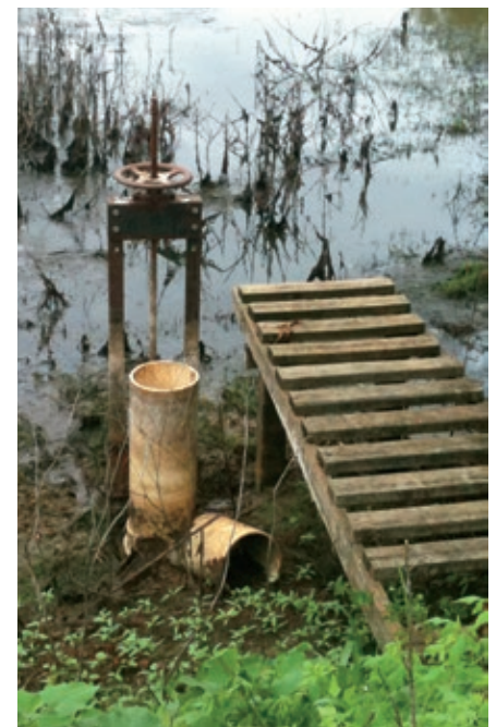
While duck ponds are drained, check and maintain water control structures to ensure they work properly. This may include replacing valves, lubricating moving parts, and removing muck.
