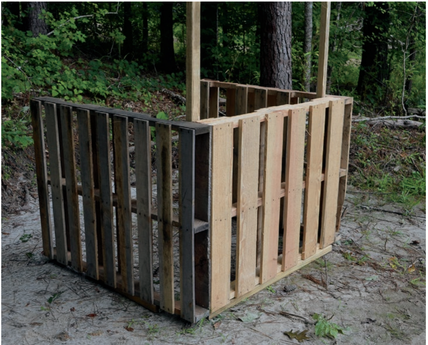
Here is an example of a one man half-height blind. This works well on an elevated platform where you don't need as much concealment. Wrap it in burlap and screw a few leafy branches to it and you'll be amazed at how well it blends with natural surroundings.
