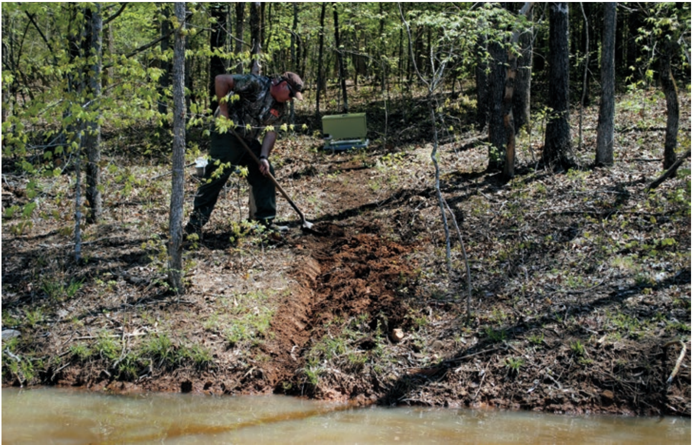
This aeration system went in the same day fish attractors were installed before the fish were stocked. The water level was at full pool flowing out the standpipe and the emergency overflow was about three feet higher; hence the aeration pump motor was installed up about six feet above the current water level.
