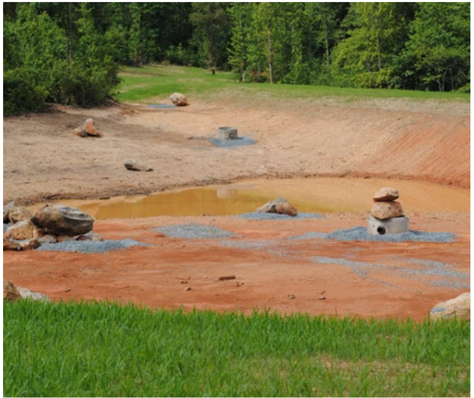
Designing and laying out this smallmouth lake required planning and knowledge of the species before the water ever started flowing. Besides rocks from the property, this landowner also incorporated man-made concrete pipes for underwater smallmouth habitat.
