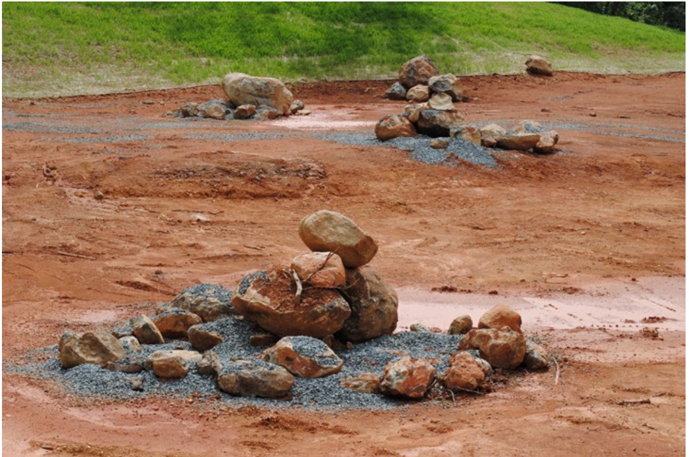
These areas provide either hiding, feeding or spawning habitat for the smallmouth bass. Things not normally found in your typical manmade pond.
