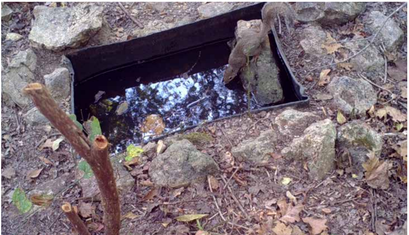
Installed "Wildlife Watering Device" looking down-slope. It is critical when installing to use a level in the bottom of the device to level the watering device so it will hold the full amount of water (27 gallons). Rocks should be placed up against the end of the device on the outside and the down slope end to assist in keeping the half barrel in place (see rocks in the picture above).
