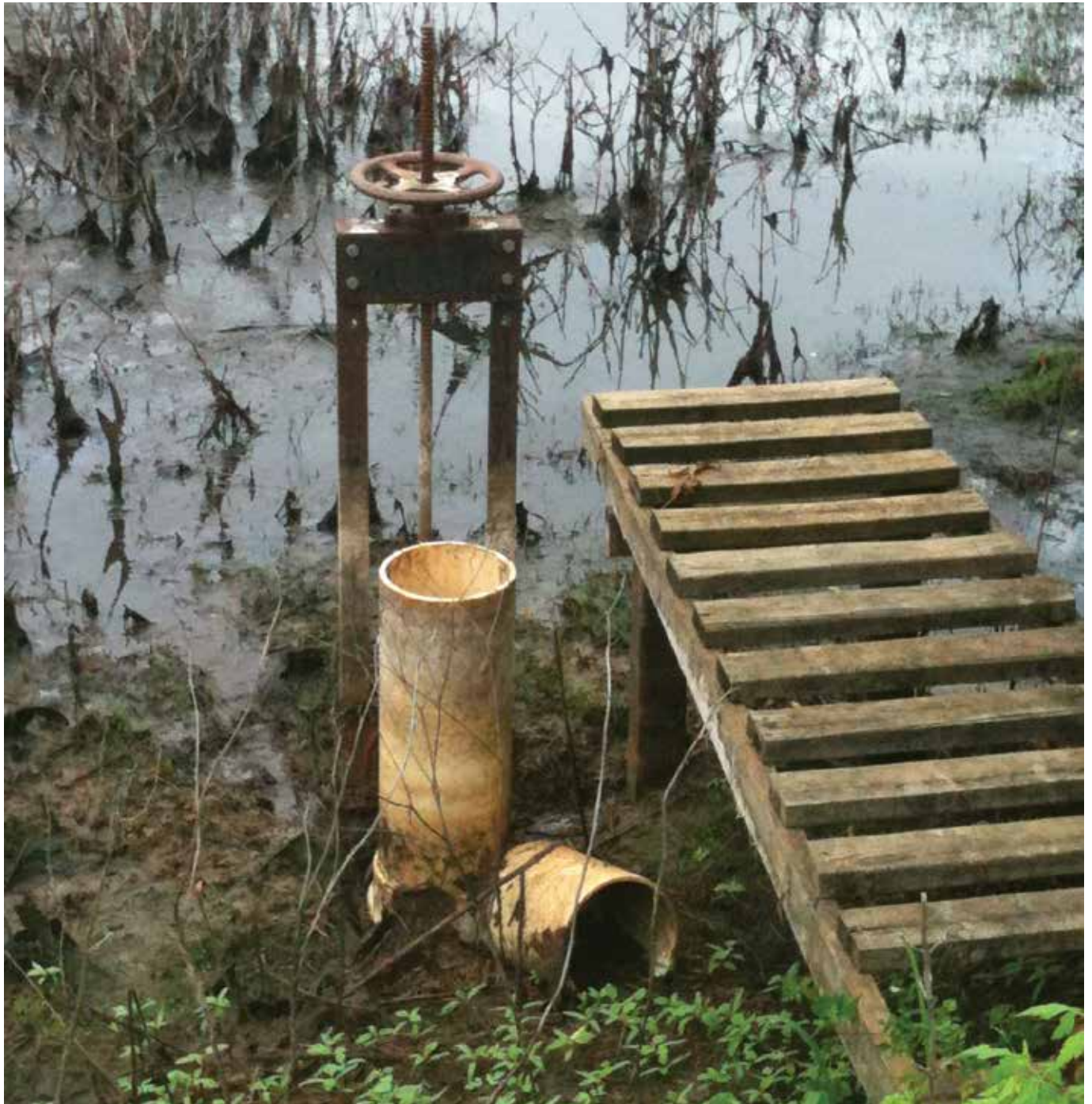
Water control structures and valves should be inspected, maintained and repaired annually.
