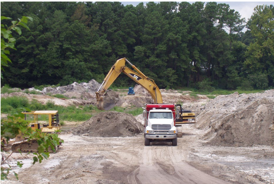
Draining, scraping and deepening your lake may be the best solution for decades or centuries of high organic build up. Although expensive, it turns succession back and will leave you with decades of worry-free lake management regarding poor water quality.
