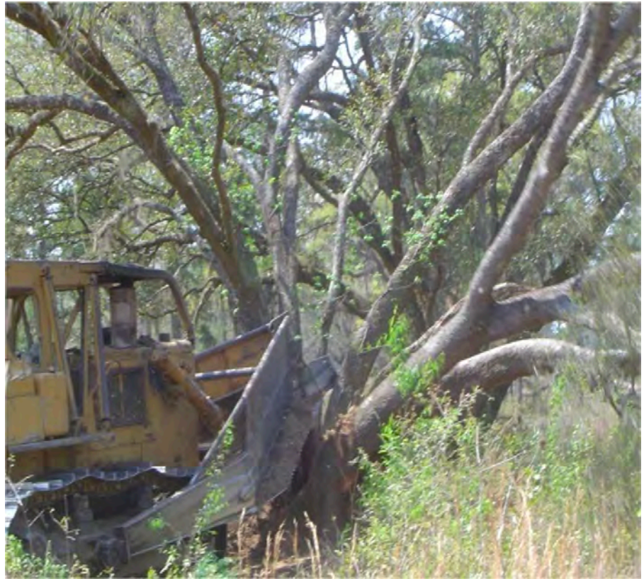
A D-8 bulldozer KG-stinger blade to split and knock down live oak trees for hardwood reduction projects. This practice can be costly ($125-150) per acre or more depending on the density of lives oaks removed.
