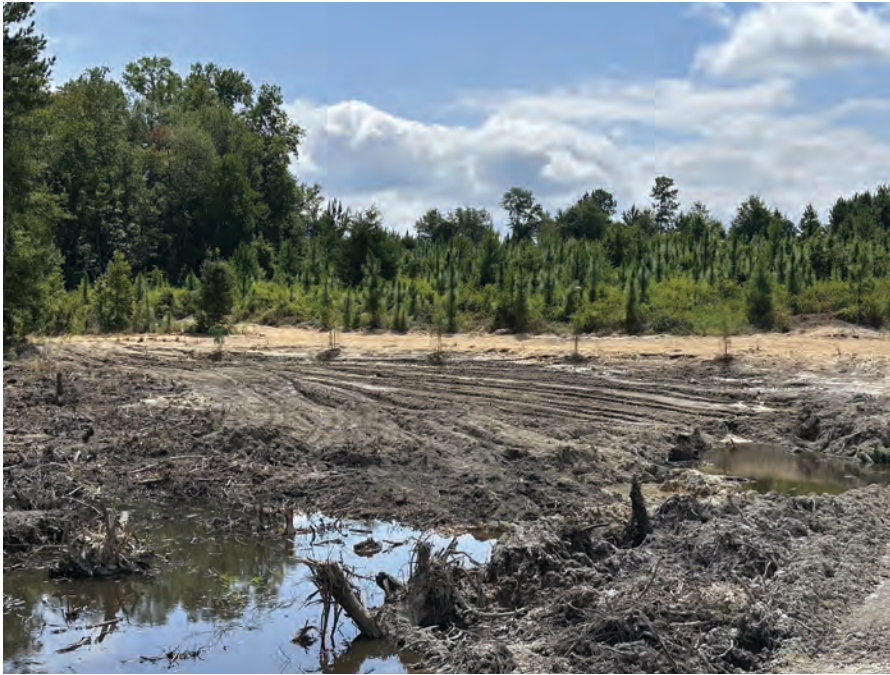
Depth, bottom contour, and shoreline slope are all important to create a waterbody that promotes a high-quality waterbody from water chemistry to the fish themselves. Photo Credit: Ryan Engel
