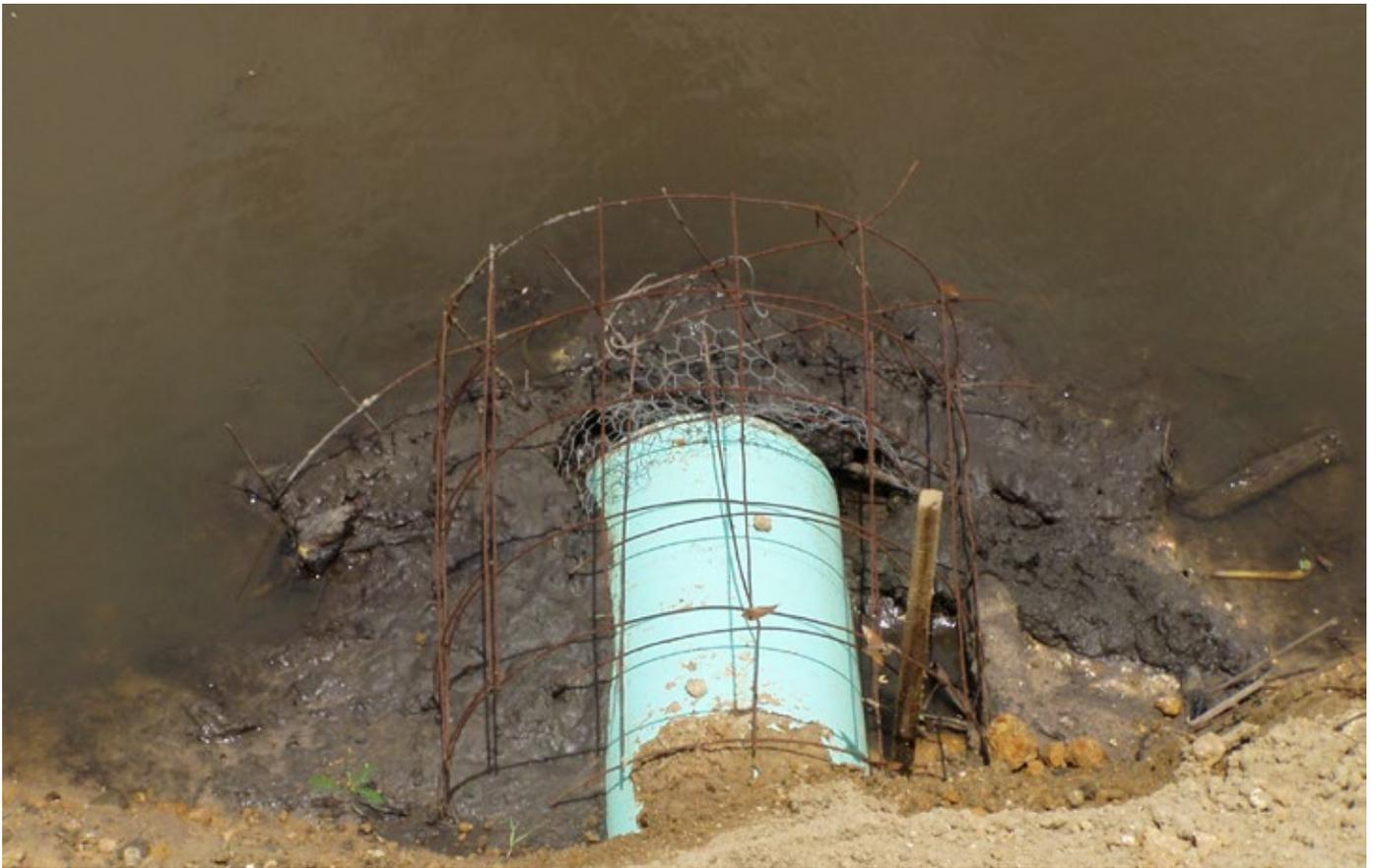
*This is a poor example of trying to keep beavers from clogging a drain.*
