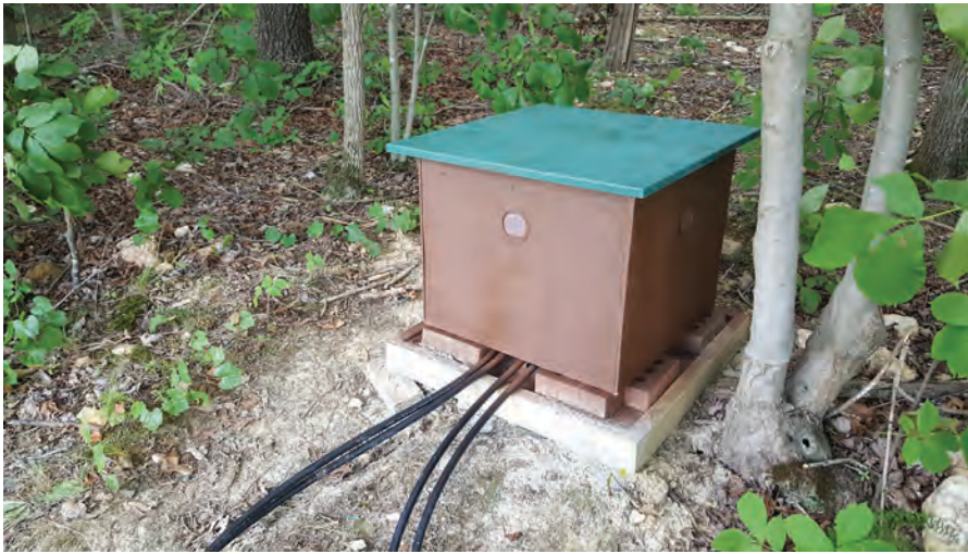
Another flood prevention measure is to make sure any aeration pumps are above any possibility of being flooded.
